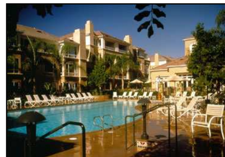
Figure 12 - "The Colony" Built in 1998, the Colony is a multifamily development in Newport Beach, CA. This development incorporates a common swimming pool and an adjacent spa into its amenity package offered to the residents. These amenities often create a standard for the competitive market area. Source: ULI: Development Case Studies
