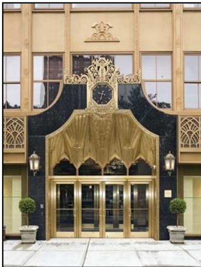
Figure 22 – “Eleven80” The “Eleven80” building was abandoned by its previous owner in the early 1980s. This art deco building presented a daunting rehabilitation task: entire floor plates had rotted, sections of the facade were crumbling, and steel beams and columns had rusted through and separated from the structure. Source: ULI: Development Case Studies
