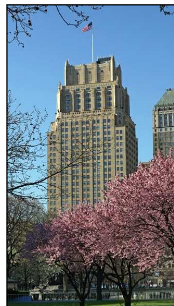
Figure 21 –“Eleven80” To finance “Eleven80” in 2007, the developer had to use seven sources of financing, one of which was the federal Historic Preservation Tax Credit program. Source: ULI: Development Case Studies
