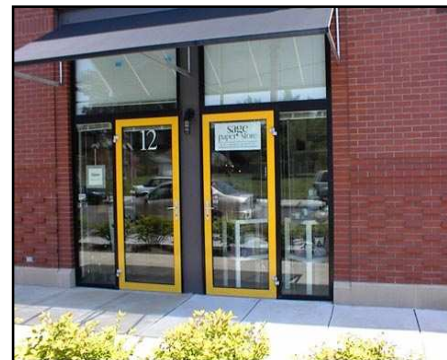
Figure 28 - "6 North Apartments" Due to the urban location, two of the three live/work units in "6 North" have been designated for commercial use. Bright yellow door frames on all ground-floor units are intended to make it easier for people with low visual acuity to locate entrances. Source: ULI: Development Case Studies
